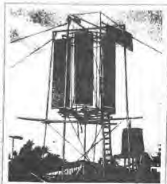
The vanes on the above vertical windmill are shaped like airplane wings to form a vacuum to generate more power.
